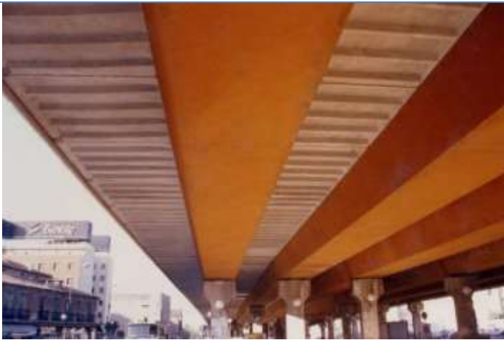
Avenida de la Albufera viaduct in the M-30. Madrid. Spain (1993)
