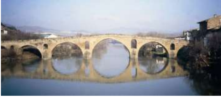
Rehabilitation of Puente la Reina bridge (S XII). Navarra. Spain (1989)
