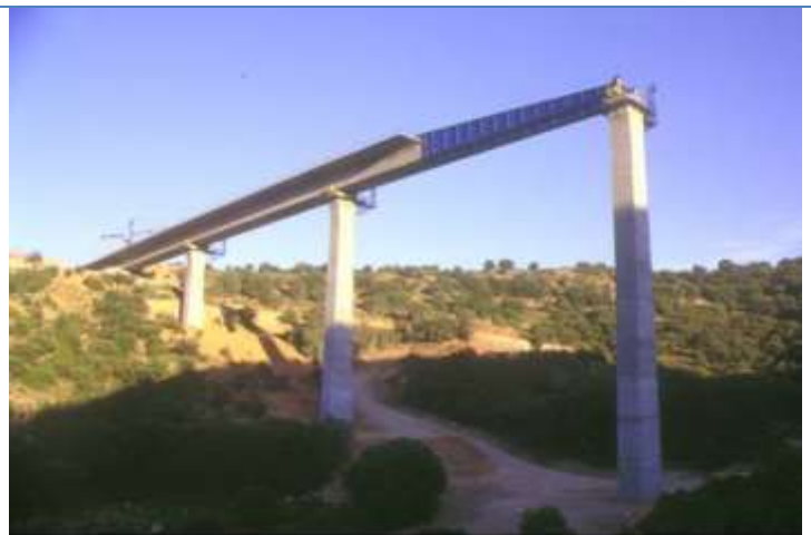
Arcos del Jalón viaduct. High speed line Madrid-Zaragoza. Spain (2006)
