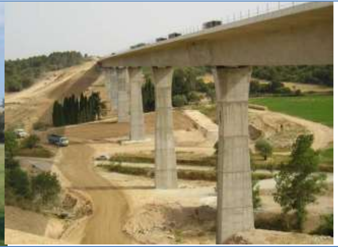
Ricardell viaduct for the high speed line Barcelona-Francia. Gerona. Spain (2007)
