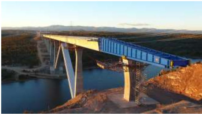
Viaduct for the high speed line over the Tera River. Zamora. Spain (2014)
