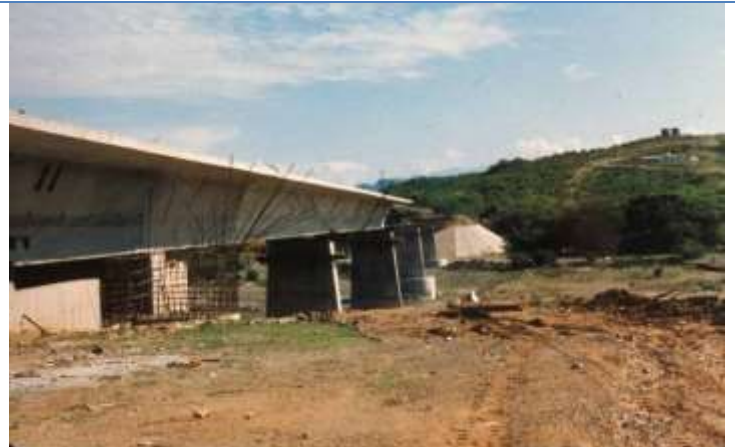
Baridaguato viaduct. Mexico (1982)
