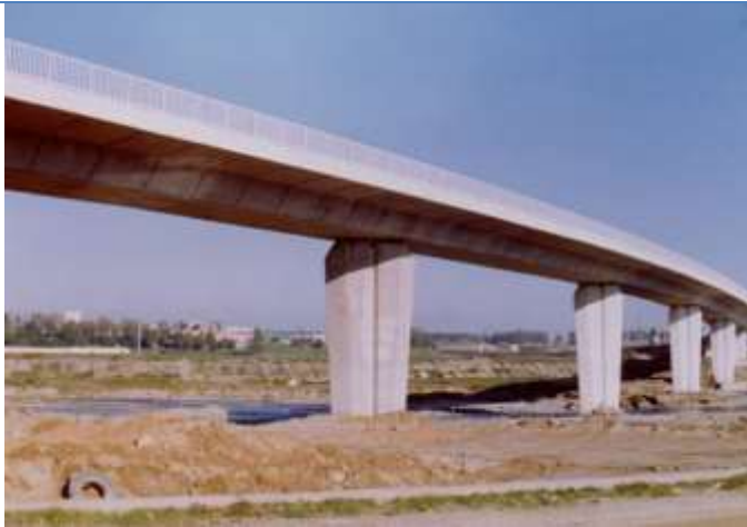
Viaduct over the Ripoll River. Barcelona. Spain (1989)
