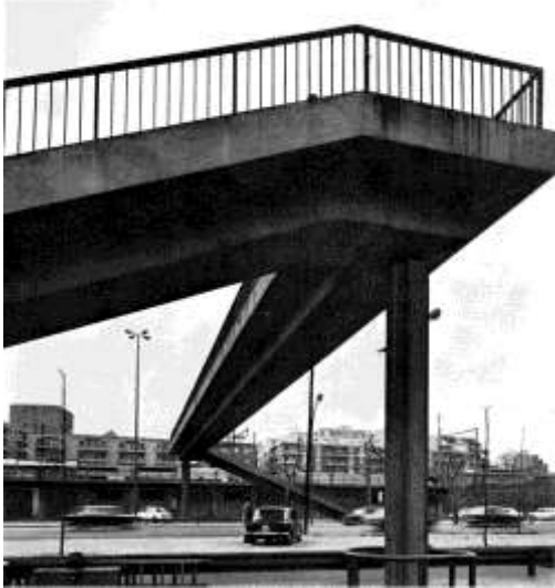
Metal footbridge. Barcelona (1973)
