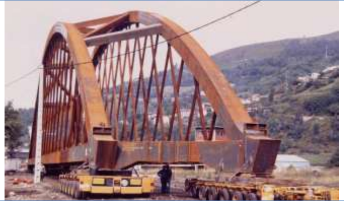
Railway bridge over the Caudal River. Asturias. España (1992)
