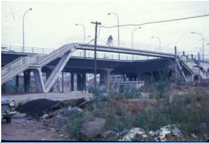
Two precast footbridges. Barcelona. Spain (1973)
