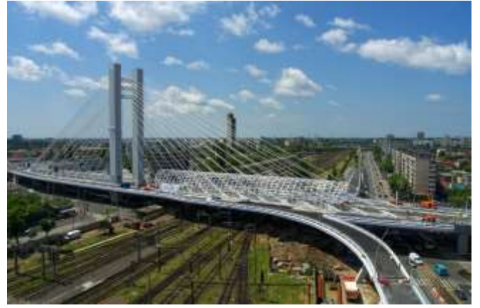
Basarab Bridge, Bucarest, Romania (2012)
