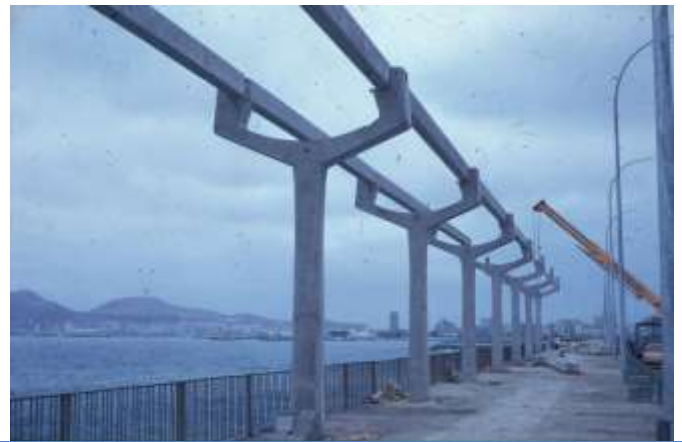
2 KM elevated railway viaduct. Santa Cruz de Campezo. Canarias. Spain (1972)
