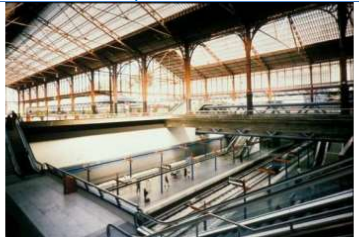
Príncipe Pío railway and Metro station. Madrid. Spain (1994) Arq: J. Casero
