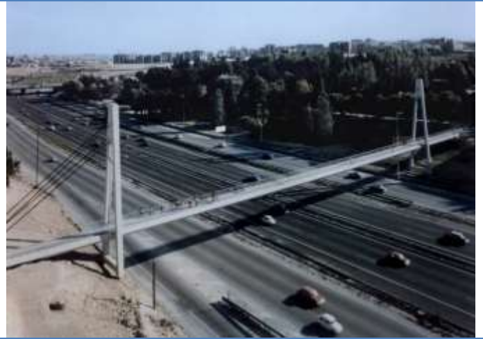
La Paz Footbridge over the M-30. Madrid. Spain (1975)
