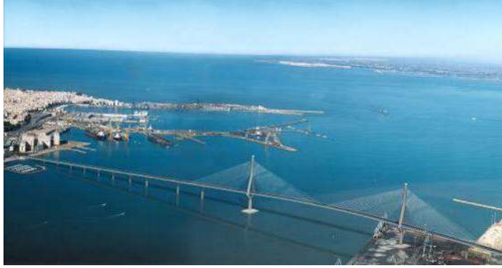
Bridge over the Cádiz harbour , Spain (under construction 2014)
