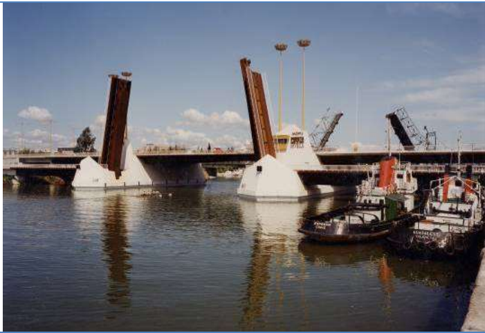
Bascule rail and road bridge over the Guadalquivir river. Sevilla. Spain (1991)
