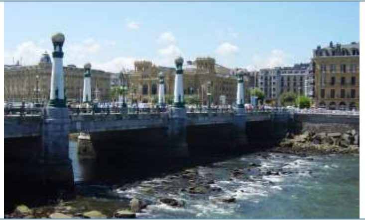
Rehabilitation of the Kursaal bridge (1912). San Sebastián. (1991)
