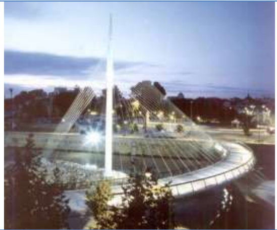
Malecón Bridge. Murcia. Spain (1996)
