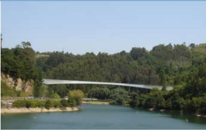
Gorostiza bridge. Vizcaya. Spain (2009)
