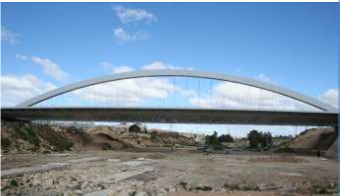
Bridge over the Vinalop3 River. Elche (2013)
