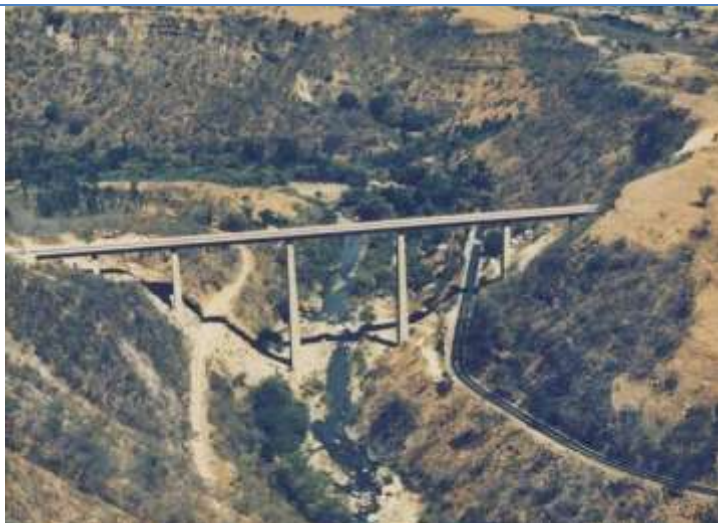
Atenquiques viaduct. Mexico (1990)
