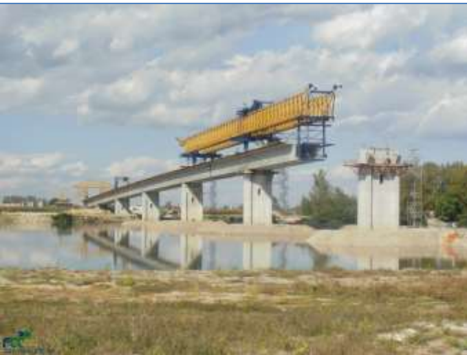
Access bridge over the Danube Bridge (2). Bulgaria (2012)
