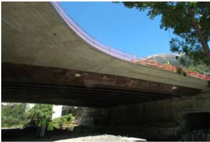
San Juliá bridge. Andorra (2010)
