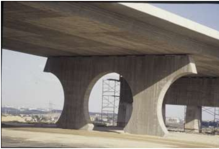
Overpass over the M-40 (3). Madrid. Spain (1994)
