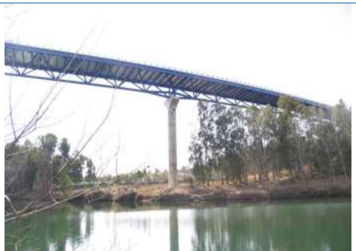
Viaduct over the Garcia Sola reservoir. Badajoz. Spain (2008)
