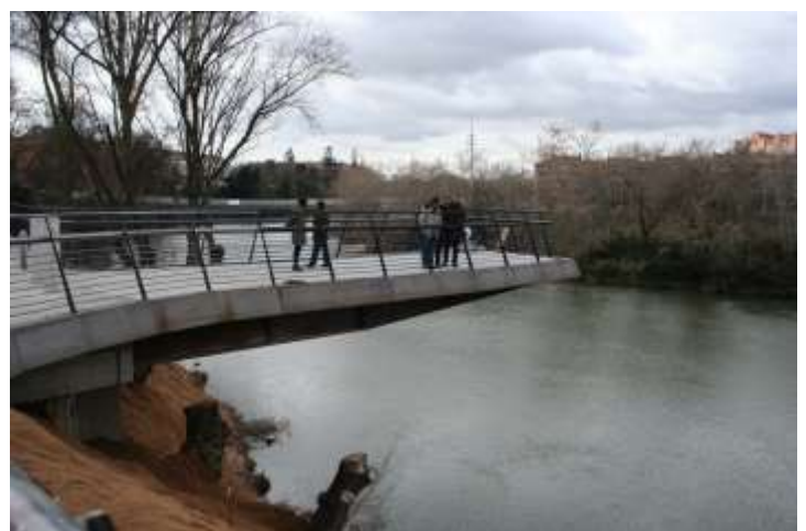
Cantilever balcony over the Pisuerga River in Valladolid. Spain (2014)
