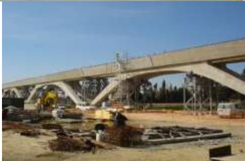
El Portal railway viaduct over the Guadalete River. Cádiz. Spain (2004)
