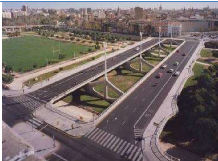
Guillem de Castro Bridge over the Turia River. Valencia. Spain (1998)
