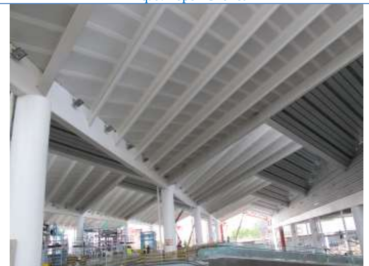
Enlargement of Atocha railway station. Madrid. Spain (2010) Arq.: R. Moneo
