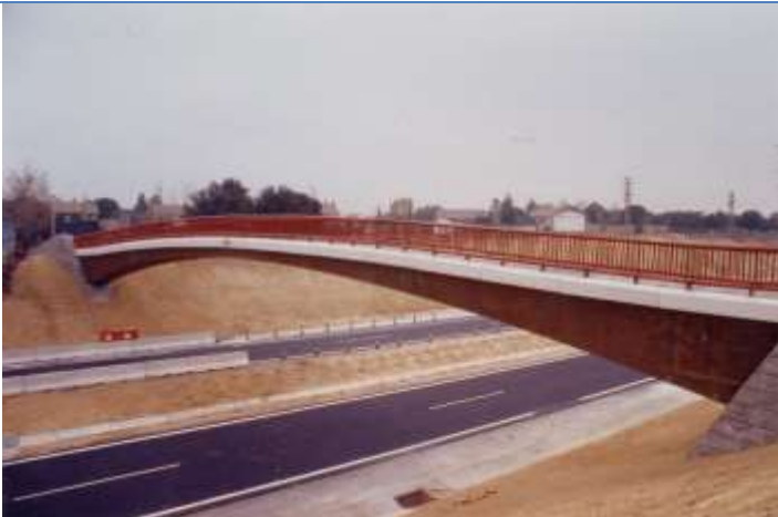
Monteclaro Footbridge over the Pinar in Majadahonda. Madrid. Spain (1994)
