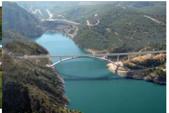
Viaduct over the Contreras reservoir for a high speed line. Cuenca. Spain (2009)
