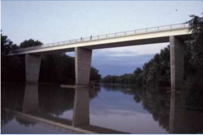
Bembezar aqueduct Sifón over the Guadalquivir River. Córdoba. Spain (1967)
