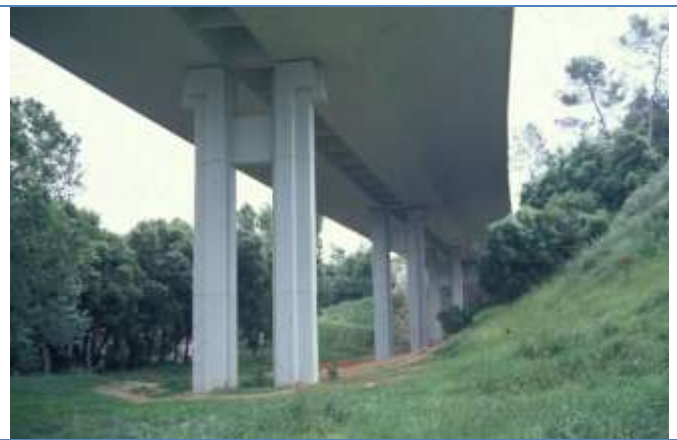
Can Ballast viaduct. Barcelona. Spain (1994)
