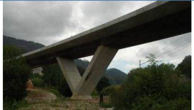
Sovilla viaduct. Cantabria. Spain (2009)
