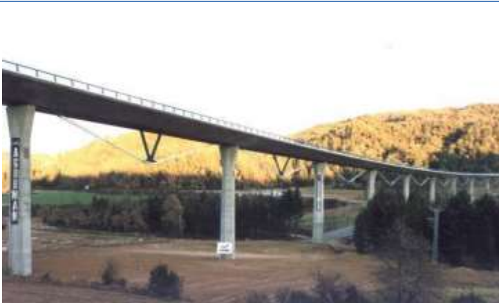
Osormort viaduct, Barcelona, Spain (1995)
