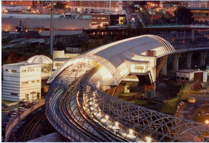
Urbinaga railway station in Vizcaya. Spain (2002)
