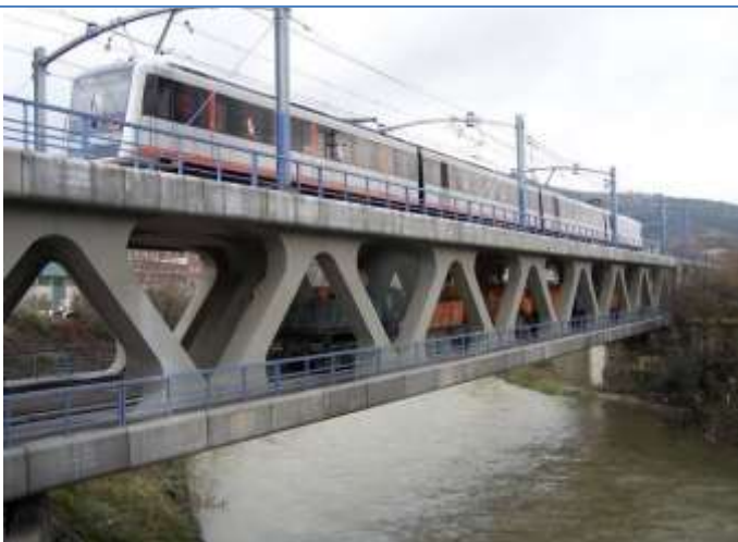
Etxebarri double level railway bridge over the Nervión River. Bilbao. Spain (2005)
