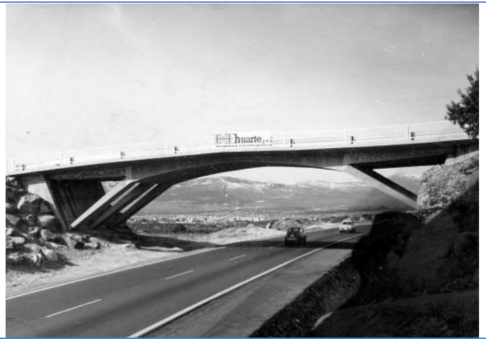
La Navata overpass
