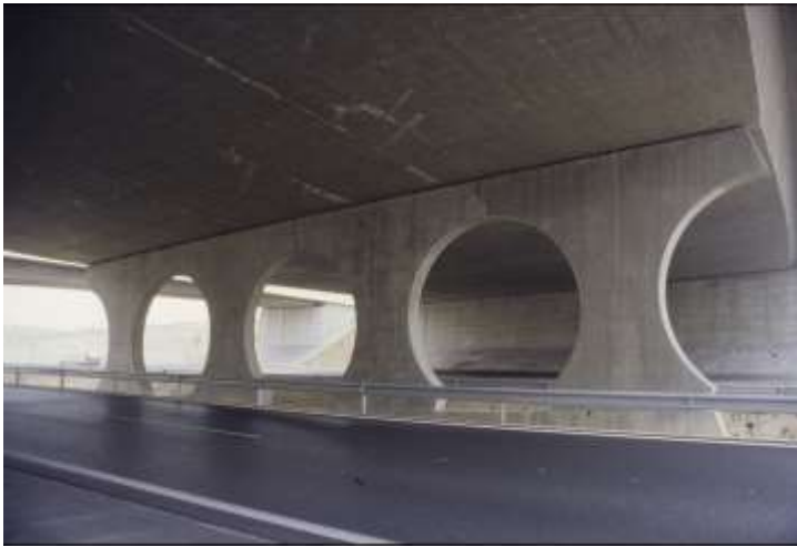
Overpass over the M-40 (1). Madrid. Spain (1994)
