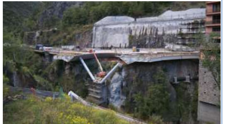
Engordany foundabout. Andorra (under construction)
