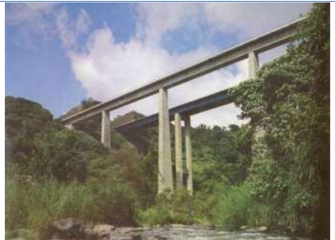
Metlac railway viaduct. Mexico (1984)
