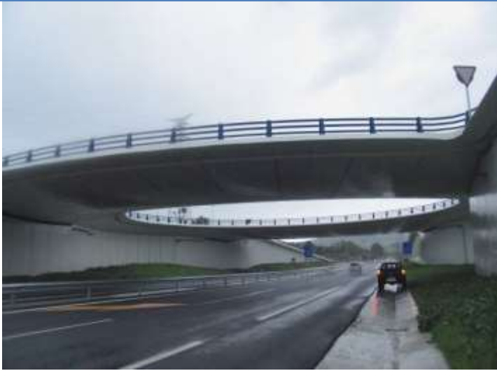
Overpass in Urnieta. Guipúzcoa. Spain (2008)
