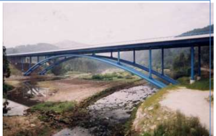
Bridge over the Escudo River. Cantabria. Spain (1999)
