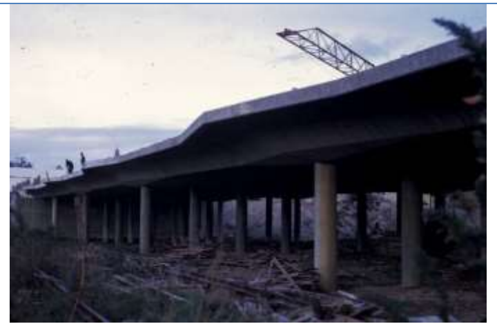
Bridge over the Tormes River. Salamanca. Spain (1970)
