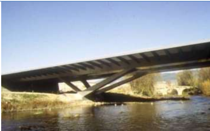
El Vergel viaduct over the Arga River. Pamplona. Spain (1997)
