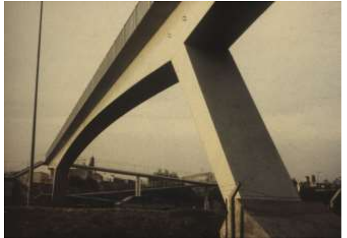
Footbridge in Buenos Aires. Argentina (1980)
