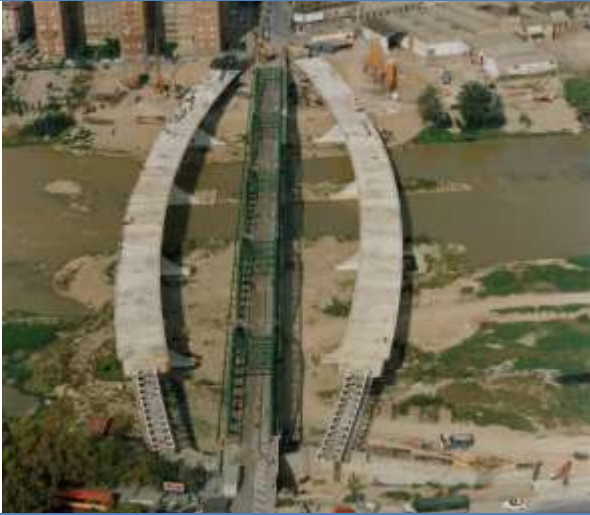
New bridge El Pilar over the Ebro River. Zaragoza. Spain (1992)
