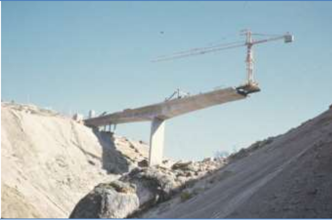
Arroyo Priego viaduct over the Iznajar reservoir. Córdoba. Spain (1968)
