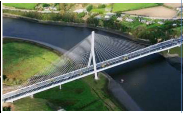
Bridge over the Suir River. Waterford. Ireland (2009)
