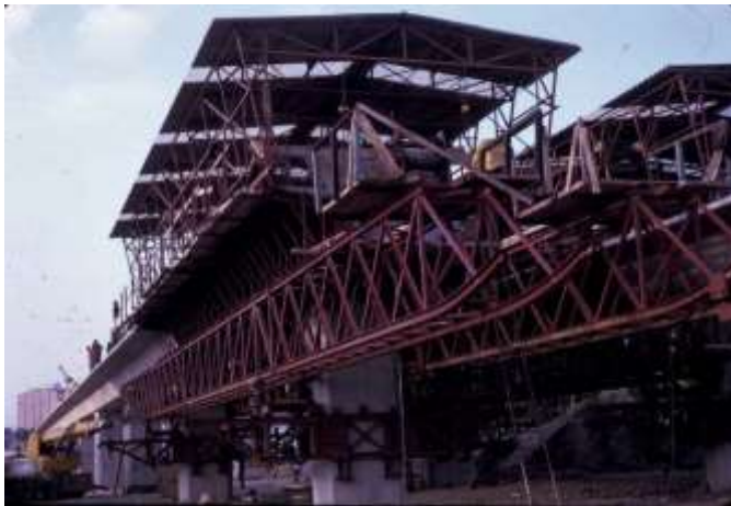
Viaduct for railway. Gerona. Spain (1972)
