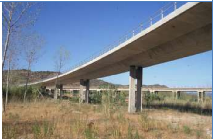
Bridge over the Siurana River. Spain (1985)
