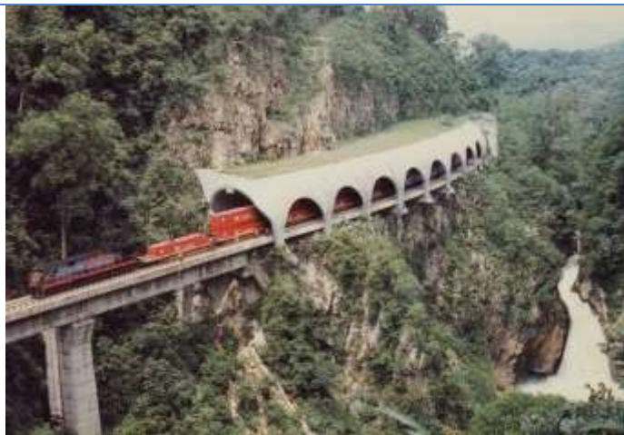
Artificial tunnel in cantilever for a railway line. Pensil . Mexico (1986)
