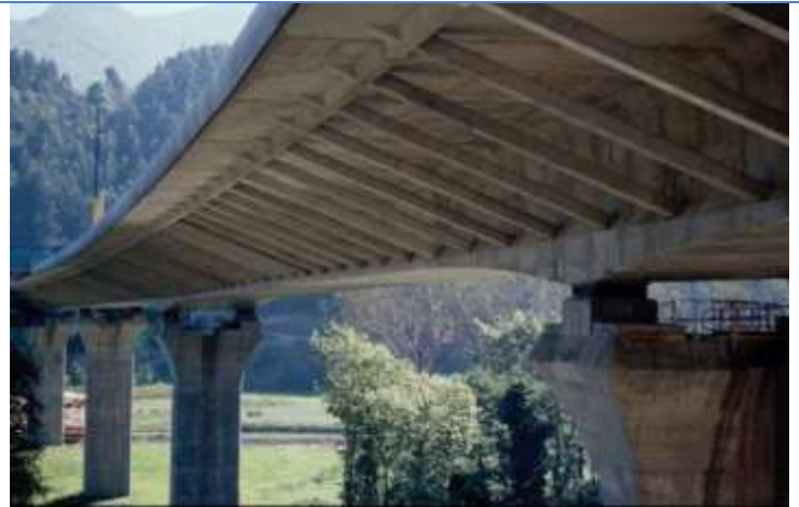
Viaduct over the Sella River. Ribadesella. Asturias. Spain (2002)
