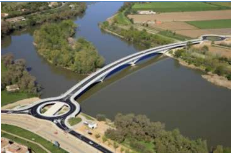
Bridge over the Duero River. Zamora. Spain (2012)
