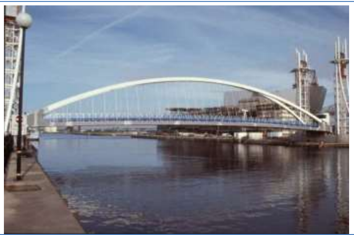
Vertical lift bowstring footbridge at Salford (Manchester). UK (1999)
