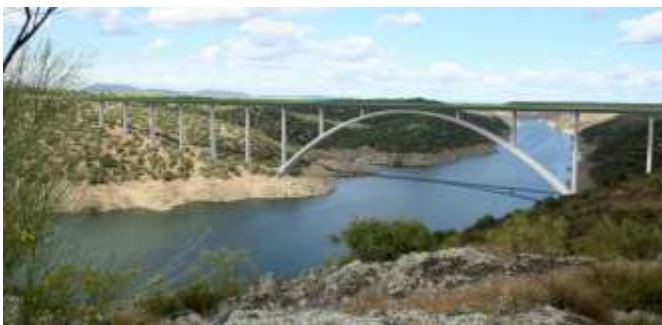
Viaduct over the Alc3ntara reservoir for the high speed line. C3ceres. Spain (under construction)
