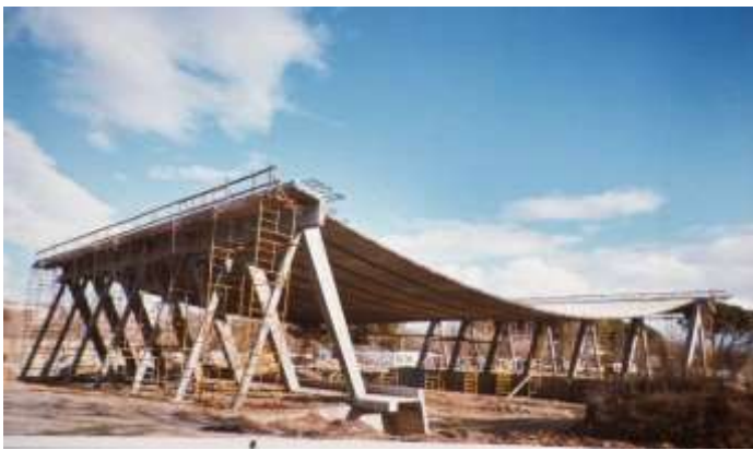
Suspended roof of Club de Campo riding school. Madrid. Spain (1968) Arq: Dominguez Salazar
