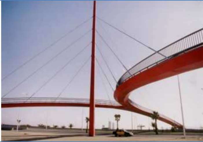
Glorias Catalanas Footbridge. Barcelona. Spain (1974)
