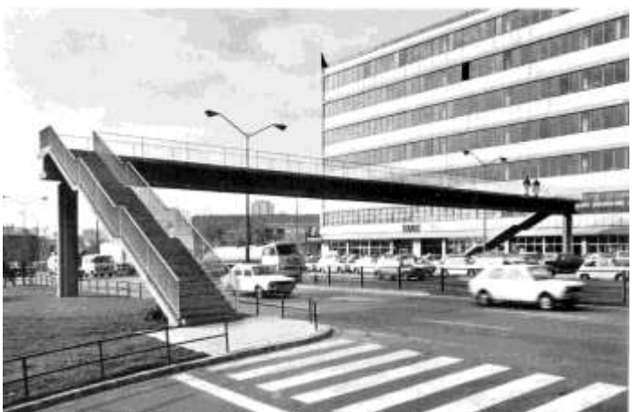
El Clot footbridge. Barcelona. Spain (1973)
