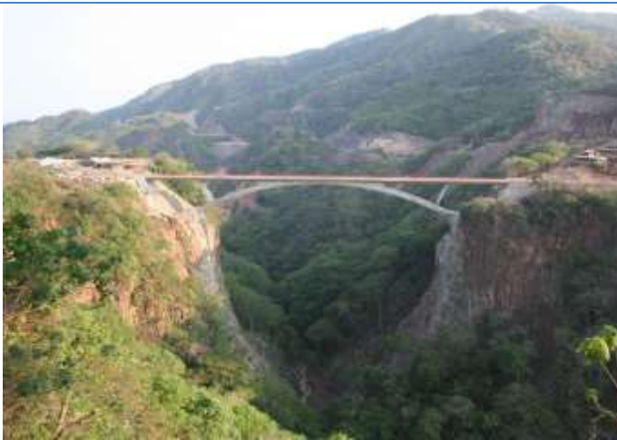
San Sebastián Bridge. Mexico (2006)
