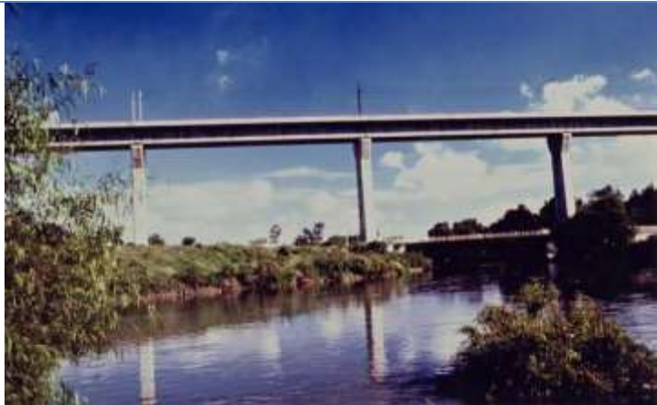
Railway viaduct over the Tula River. Mexico (1980)
