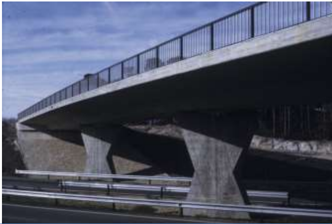
Overpasses in Barcelona–La Junquera Highway. Spain (1970)
