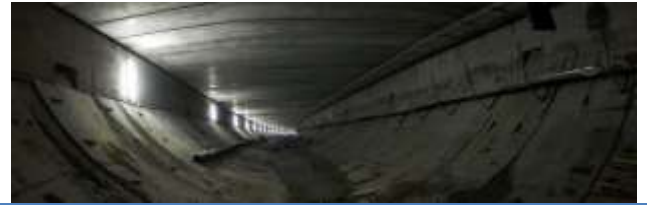
Prestressed concrete slab in the M-30 tunnels . Madrid. Spain (2008)
