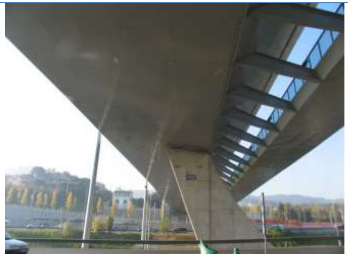
Congost overpass in the A-2. Barcelona. Spain (2008)
