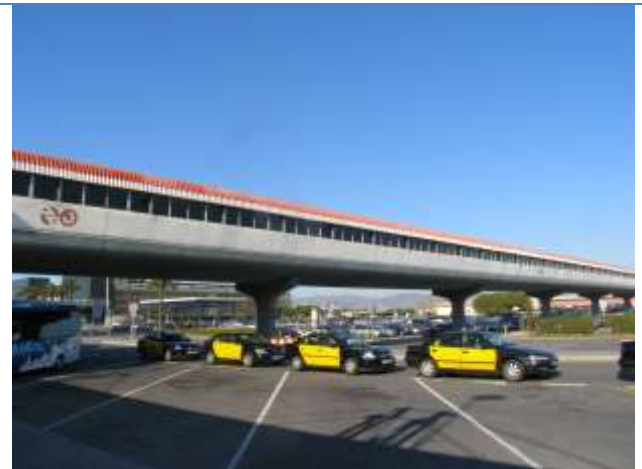
Sans Airport footbridge. Barcelona. Spain (1974)
