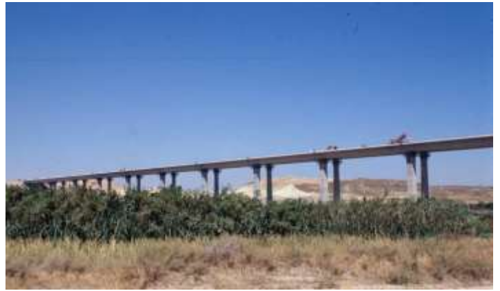
Viaduct over the Huerva river. High speed line Madrid-Zaragoza. Spain (2006)
