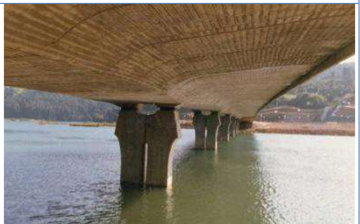
Bridge over the Plentzia River. Vizcaya. Spain (1993)
