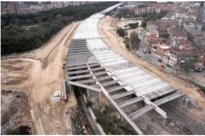
Railway cover in Villaverde . Madrid. Spain (2007)
