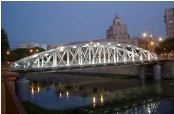
Rehabilitation and strengthening of the Puente de Hierro (S XIX). Murcia. Spain (2004)
