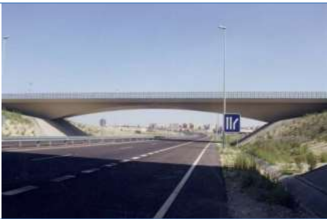
Overpass in the Coslada transport centre. Madrid. Spain (1994)
