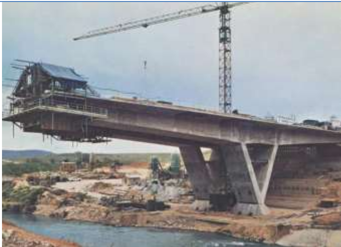
Bridge over the Júcar River. Cuenca. Spain (1977)
