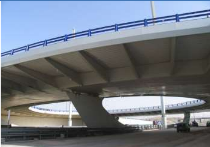
Viaduct over the M-45. Madrid. Spain (2003)
