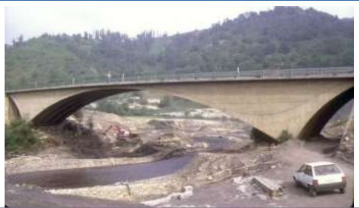
Bridge over the Caudal River. Mieres. Asturias. Spain (1968)
