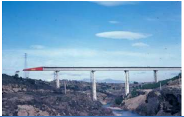
Alcanadre aqueduct. Huesca. Spain (1977)
