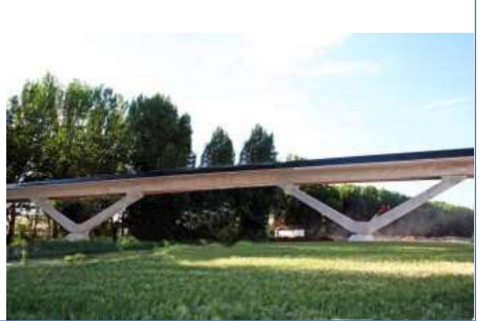
Viaduct over the Júcar River. Cuenca. Spain (2009)
