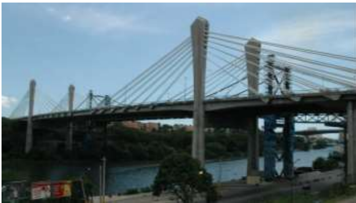
Bridge over the Ozama River. Dominican Republic (2000)
