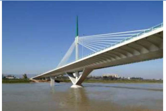
Andalucía Bridge over the Guadalquivir River, Córdoba, Spain (2005)
