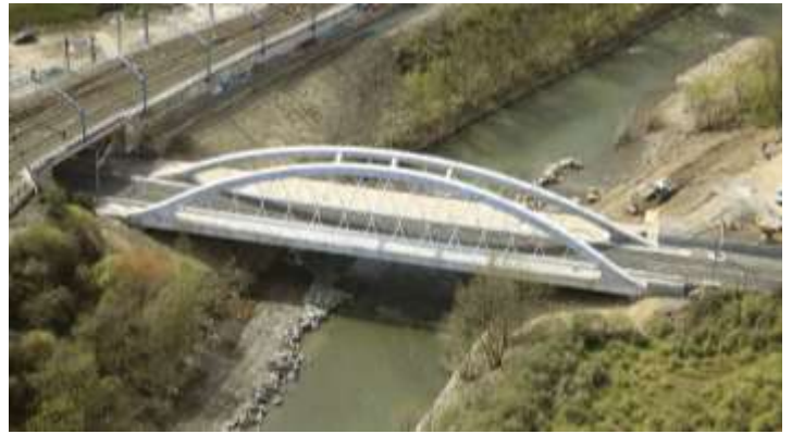
Railway bridge over the Nervi3n River. Vizcaya. Spain (2012)
