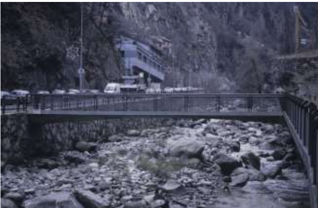
Footbridge in Andorra (1995)
