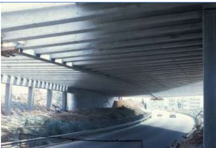
Glorias Catalanas square underpass. Barcelona. Spain (1974)
