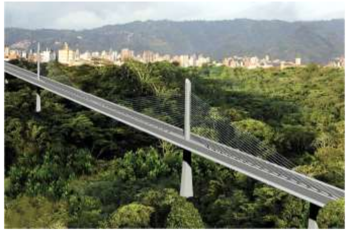
Carrera Novena viaduct in Bucaramanga. Colombia (under construction 2014)
