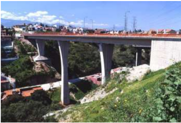
Huixquilucan viaduct. Mexico (1997)
