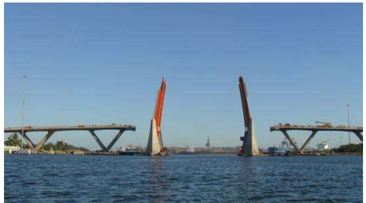
Albatros bascule bridge. Mexico (2009)
