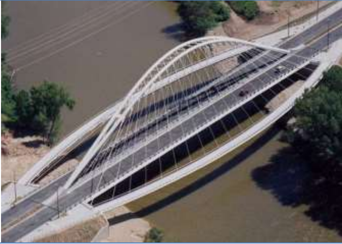
Bridge over the Ebro River. Logroño. Spain (2003)
