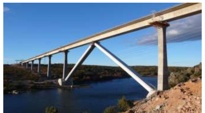
Viaduct over the Tera River. Zamora. High speed line Madrid-Galicia. Spain (2014)
