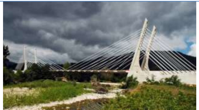
Bridge over the Besaya River. Cantabria. Spain (2009)
