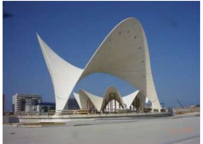
HYPAR concrete shell in the Oceanographic Park. Valencia. Spain. (1999) Based on a Félix Candela idea
