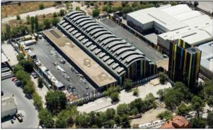
Rehabilitation Nave Boetticher (1950). Madrid. Spain (2011)
