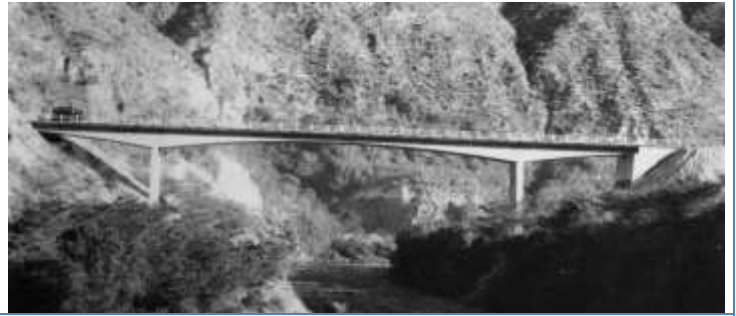
Bridge over the Guayabamba River. Ecuador (1975)
