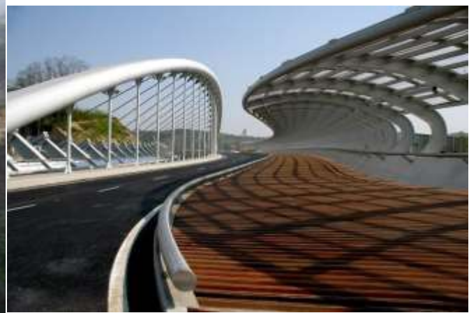
Carmen Galindo Bridge over the Galindo River. Vizcaya. Spain (2008)
