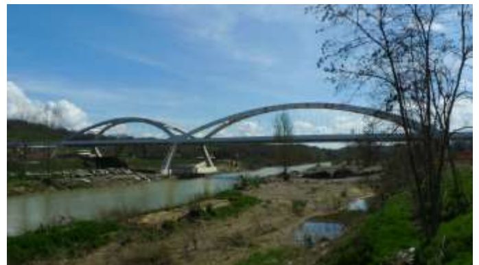
Bridge over the Arno River. Arezzo. Italy (2013)
