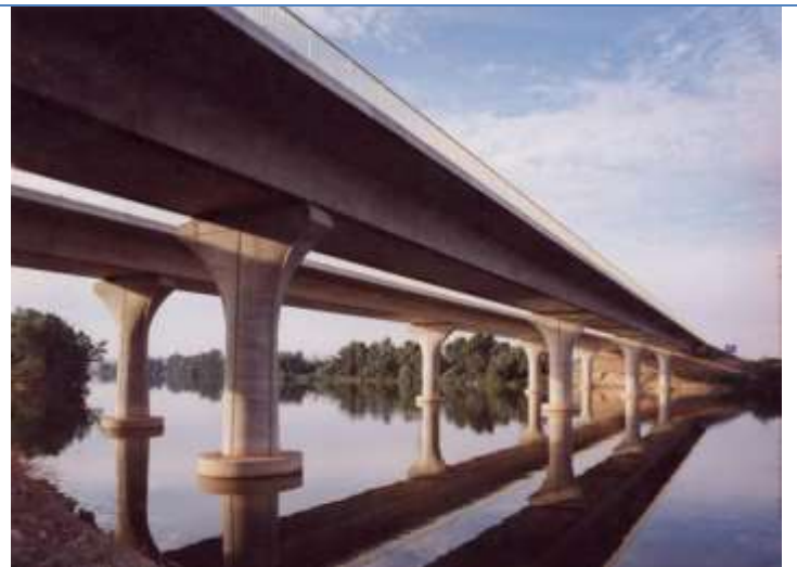
Tordesillas Bridge over the Duero River. Valladolid. Spain (1991)
