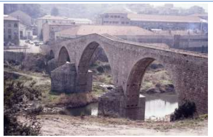
Rehabilitation of Castellbell y el Vilar bridge over the Llobregat River (S XIII)
