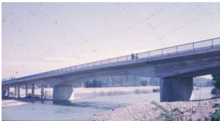
Caparroso Bridge. Navarra. Spain (1988)
