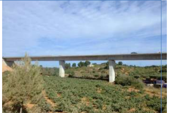
Rodenillo viaduct for the high speed line Madrid-Valencia. Cuenca. Spain (2008)
