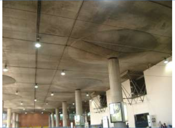
Enlargement of Atocha railway station. Madrid. Spain (2003) Arq. R. Moneo
