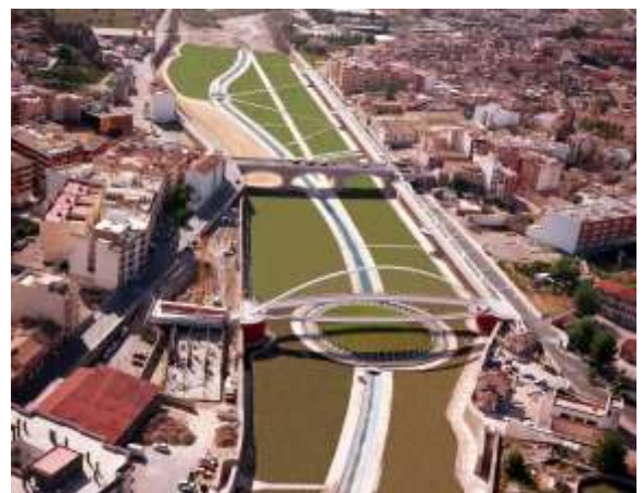
Cantilever pass over the Guadalentín River. Lorca. Spain (2002)
