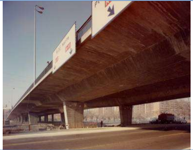
San Isidro bridge over the Manzanares River and the M-30. Madrid. Spain (1974)
