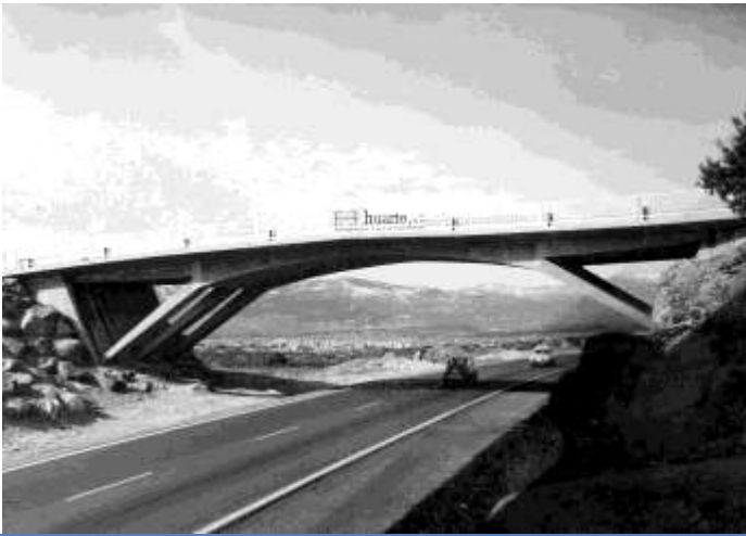
La Navata overpass (1968)
