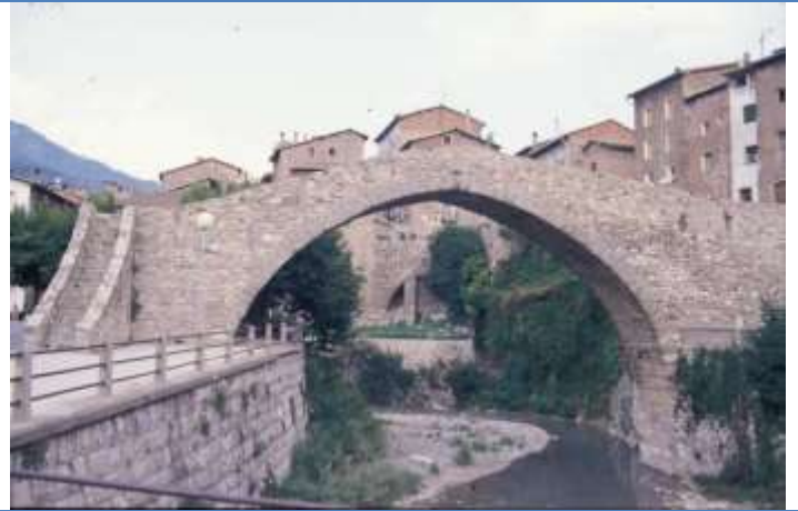
Rehabilitation of Pobla del Lillet bridge (S XIII)
