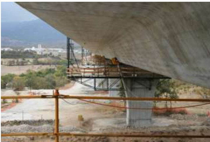
Majalahita viaduct. High speed line Madrid-Valladolid. Spain (2006)
