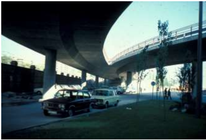
Bridge access to the Chamartín railway station. Madrid. Spain (1974)
