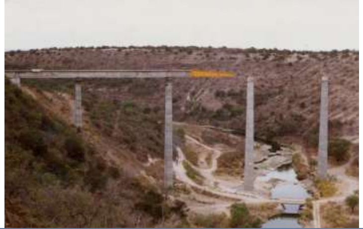
San Juan viaduct. Mexico (1993)
