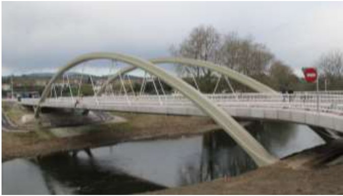
Bridge over the Saja River. Santander. Spain (2010)
