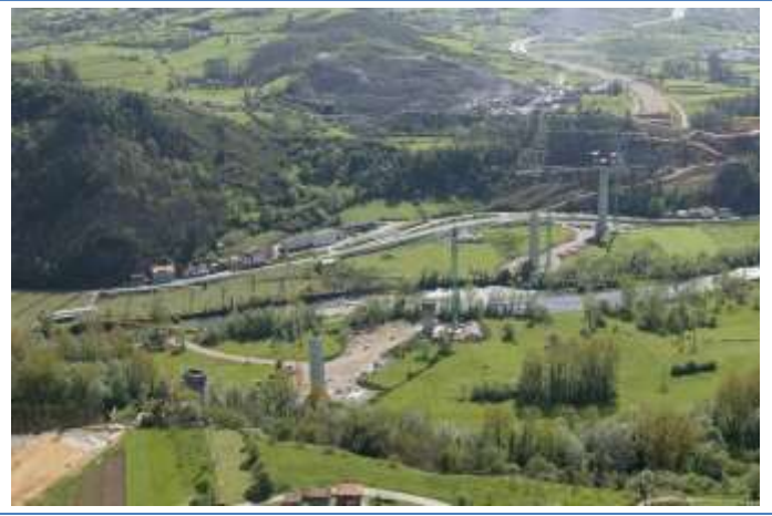
Viaducto over the Narcea River. Asturias Spain (under construction)
