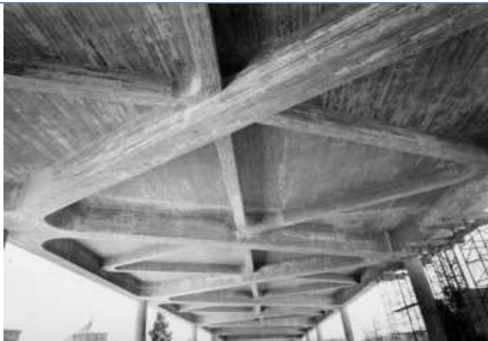
Mauricio Legendre overpass. Madrid. Spain (1976)
