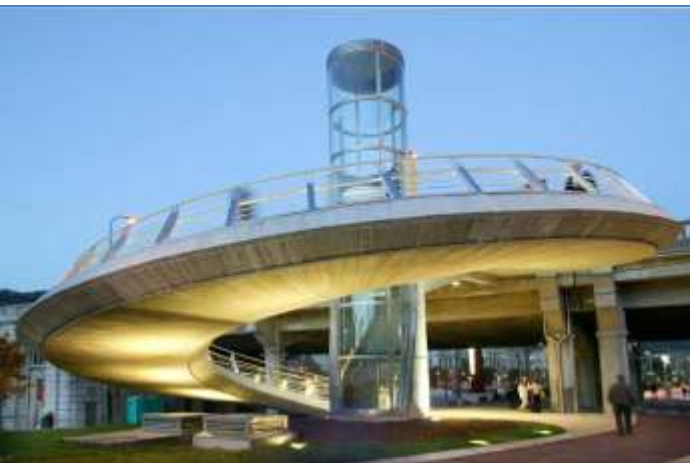
Helicoidal stairway in light concrete in Bilbao. Spain (2002)
