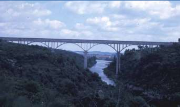
Valdeobispo Aqueduct over the Alagón River. España (1964)
