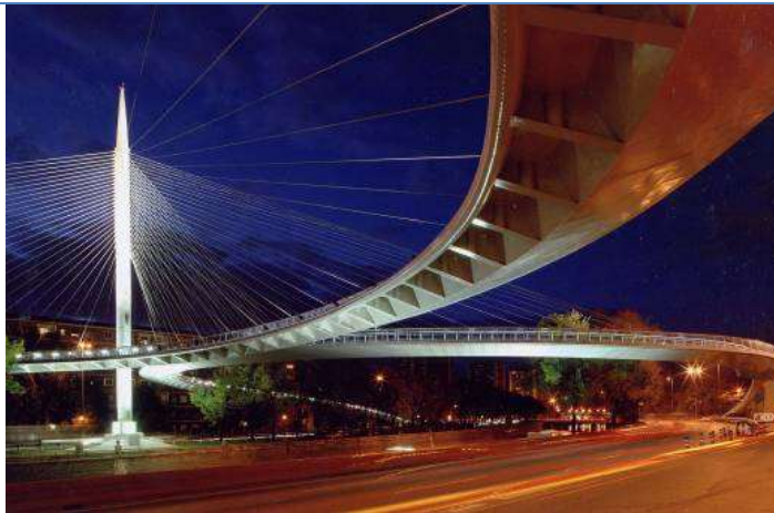
Footbridge over the M-30 . Madrid. Spain (2003)
