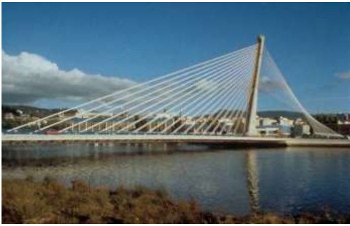
Bridge over the Lérez River. Pontevedra. Spain (1995)
