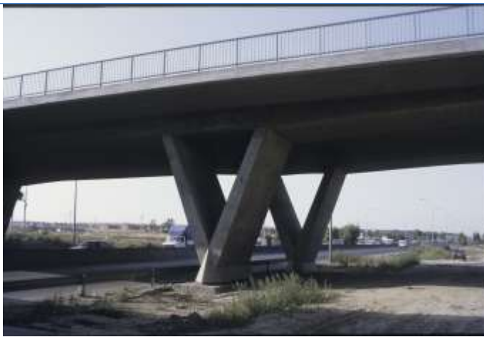
Overpasses in the Toledo road over the Culebro . Madrid. Spain (1990)
