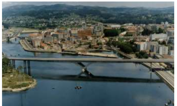
Viaduct over the Pontevedra stuary. Spain (1992)
