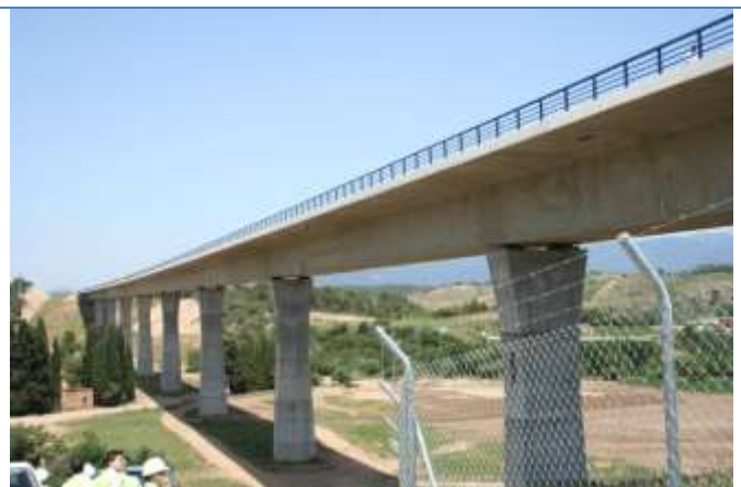
Viaduct A Muga. Gerona. Spain (2007)
