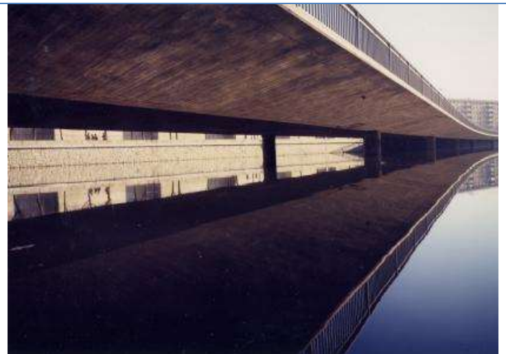
Oblicuo Bridge over the Manzanares River in the M-30. Madrid. Spain (1974)
