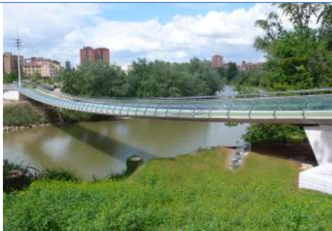
Footbridge over the Pisuerga River in Valladolid. Spain (2009)
