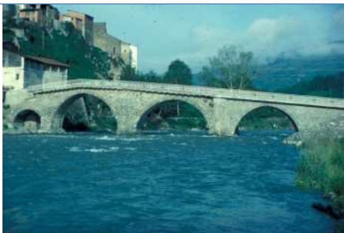
Rehabilitation of Arfá bridge over the Segre River (S XIII)
