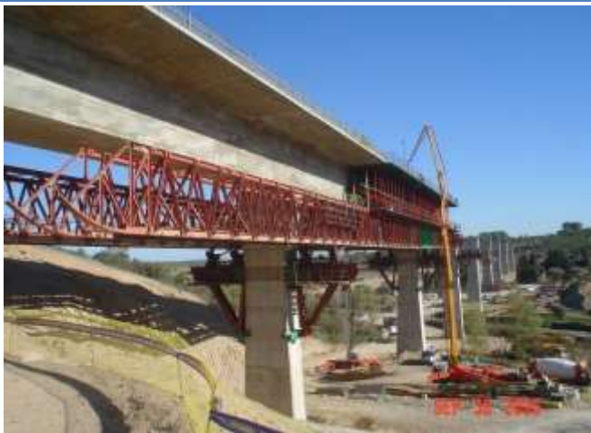
Figueras-Perpignan Viaduct. Gerona. Spain (2003)
