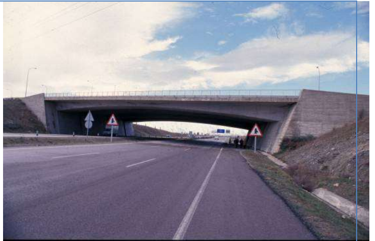
Arroyo Culebro overpass. Madrid. Spain (1990)
