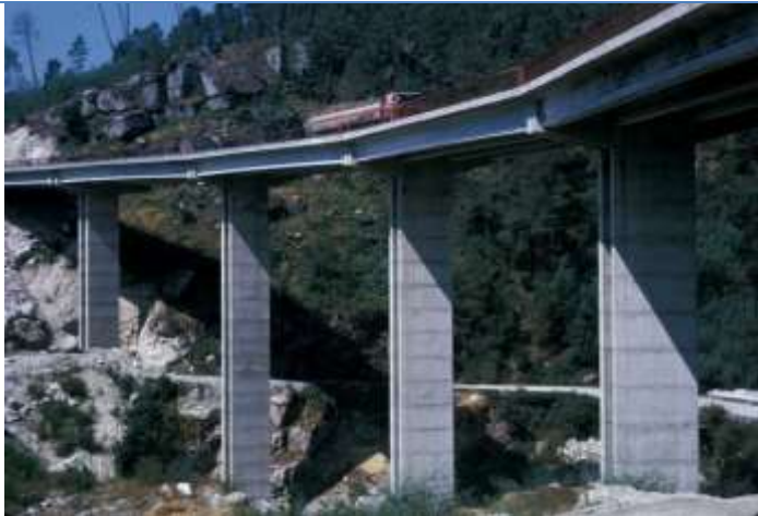
Valdepereira viaduct. Orense. Spain (1970)
