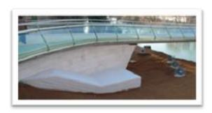
The bridge was paved using a flexible colored rubber-based solution -similar to the material used for athletic tracks with partially recycled components- extremely comfortable to walk on.
