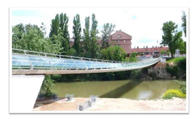
e-mail: <a href="mailto:cfcsl@cfcsl.com">cfcsl@cfcsl.com</a> www.cfcsl.com The cross section width is 5.0 m to allow for a 2.50 m pedestrian walk and a 1.50 cycle lane.
