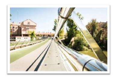
Given the uniqueness of the footbridge and the interest of the Valladolid City Council in obtaining an outstanding work, it was complemented using exquisitely designed finishing: glazed, stainless steel railings and abutment wall cladding with white limestone.
