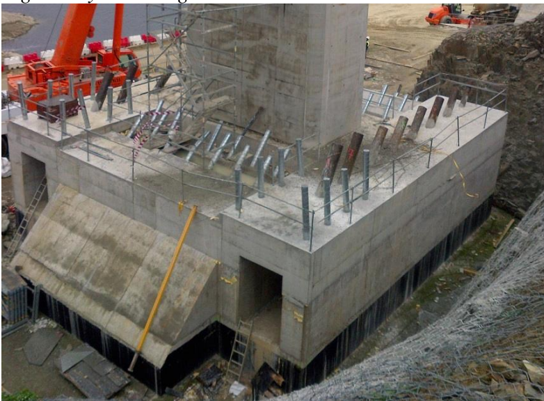
Fig 10. Stay anchorage in foundations
