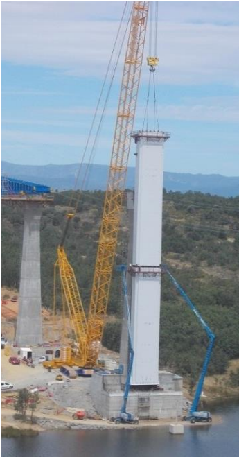
Fig. 10. Vertical erection of the semi arch
