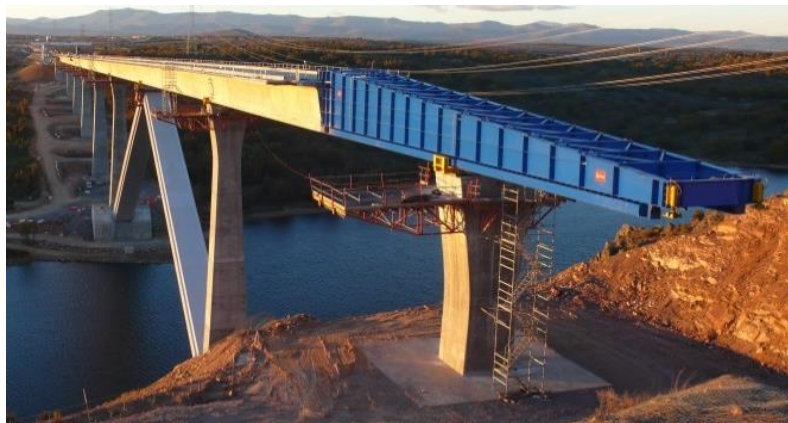
Fig. 9. Launching nose
