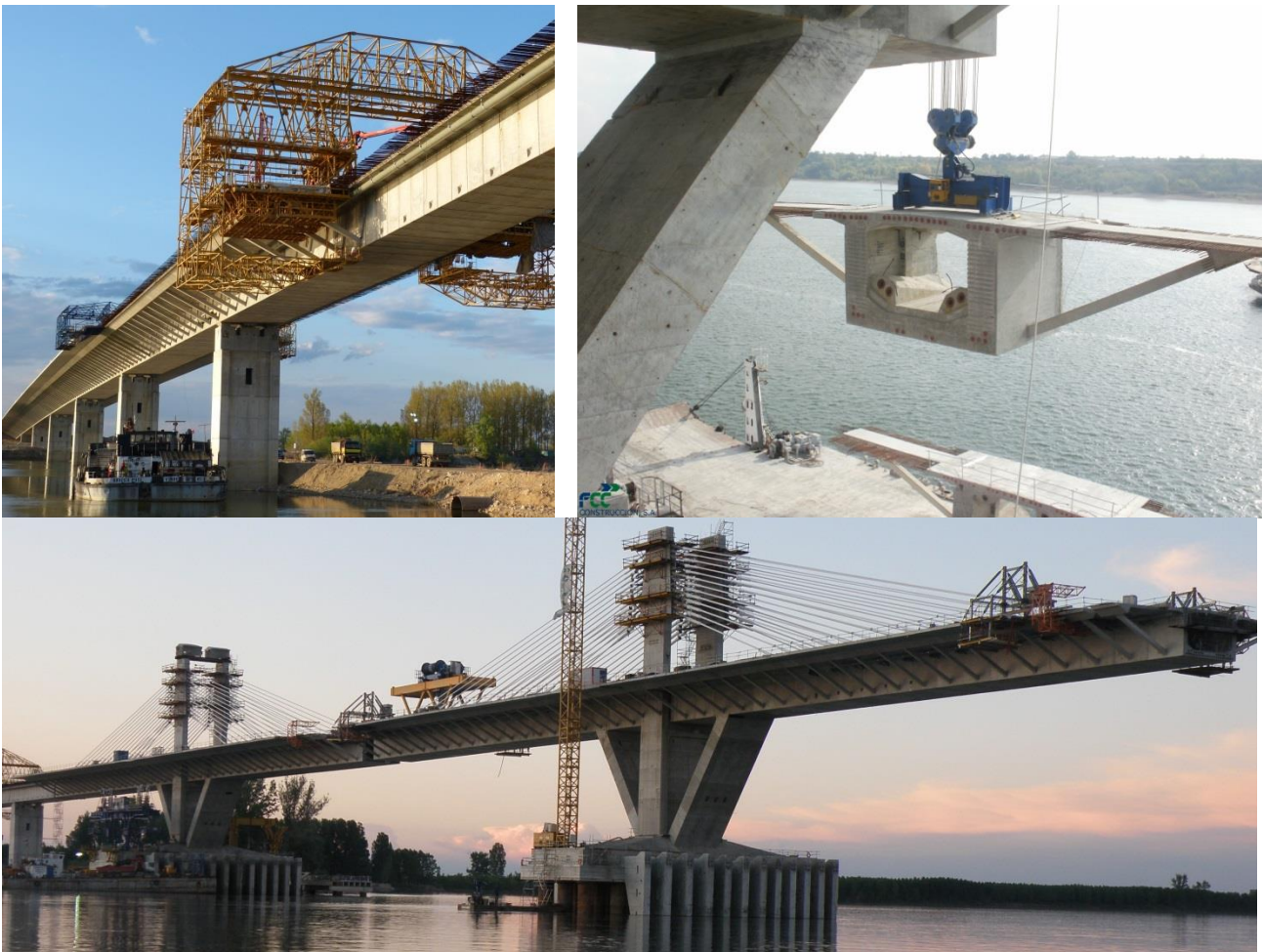
Figure 3. Construction of the main river bridge, both 80 m and 180 m deck
