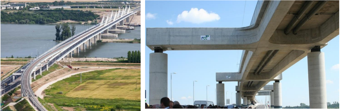
Figure 5. Elevation and final view of the 40 m railway approach bridge
