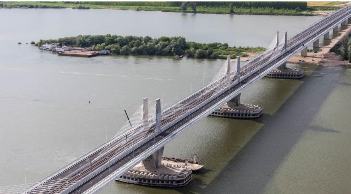
Figure 2. Main river bridge definition and final view
