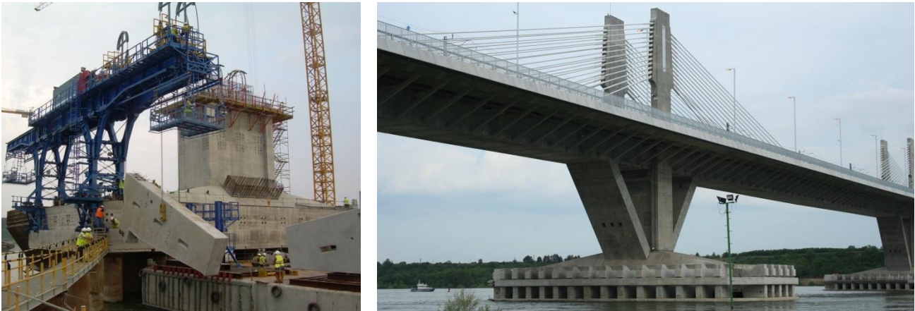
Figure 4. 180 m main river bridge foundations and ship impact protections
