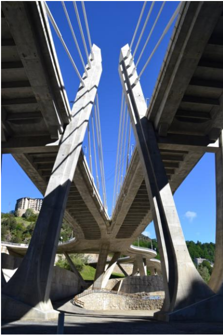
Fig. 5. Structure 1. Lower view of the bridge
