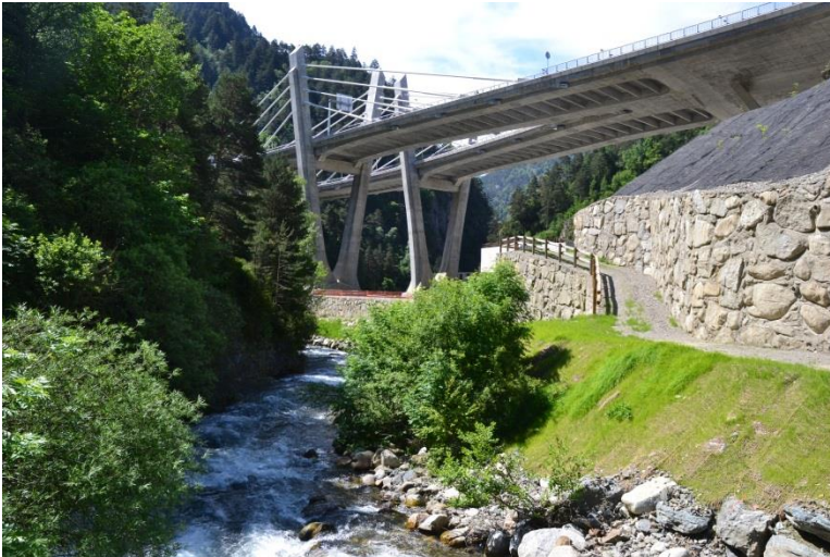
Fig. 1. View of the Structure 1
