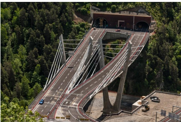
Fig. 4. View of the structure 1
