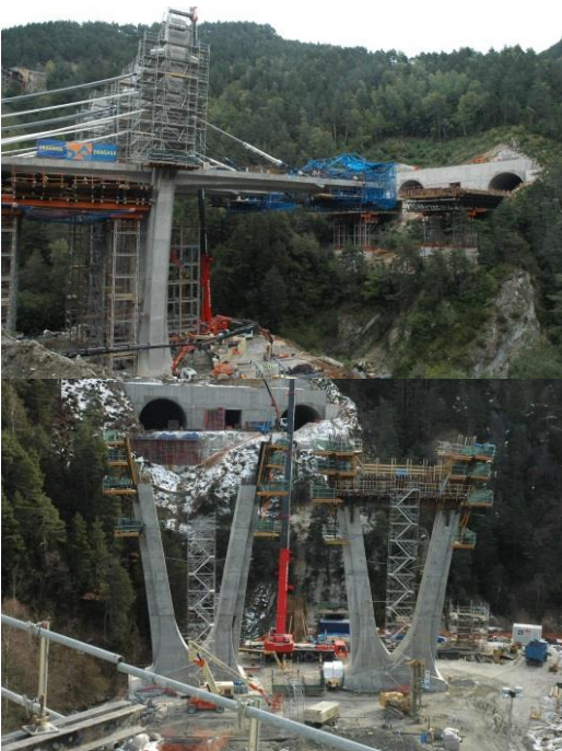
Fig. 10. Construction of Structure 1
