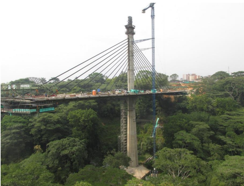
Fig. 10. Cantilever under construction
