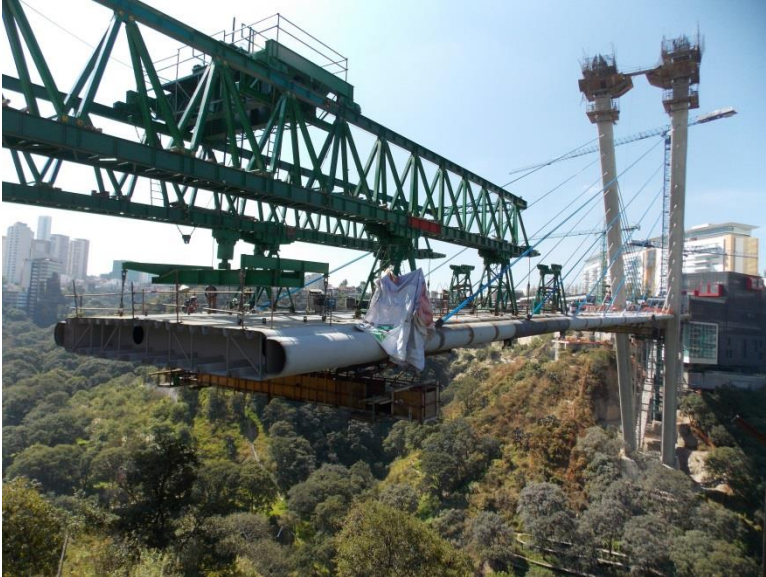
Fig. 5. Bridge under construction. Steel deck
