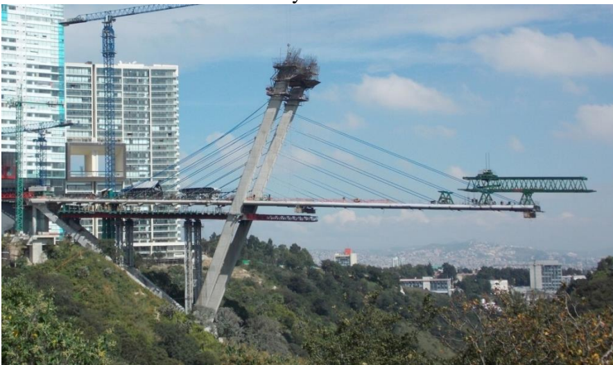
Fig. 7. Bridge under construction
