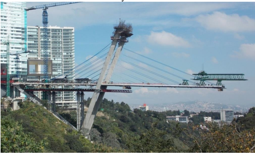
Fig. 7. Bridge under construction
