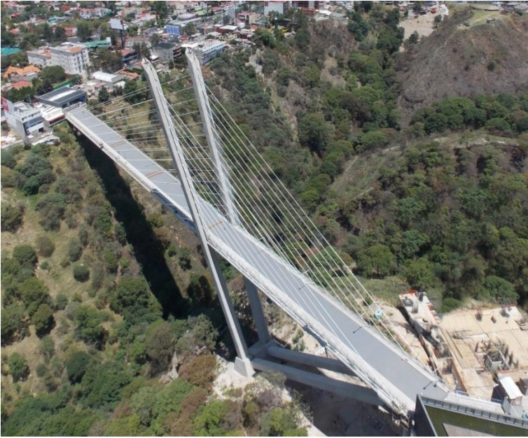
Fig. 2. Upper bridge view
