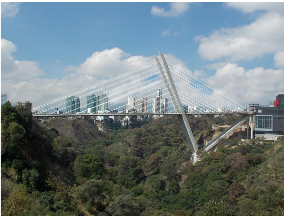
Fig. 1. General view of the bridge
