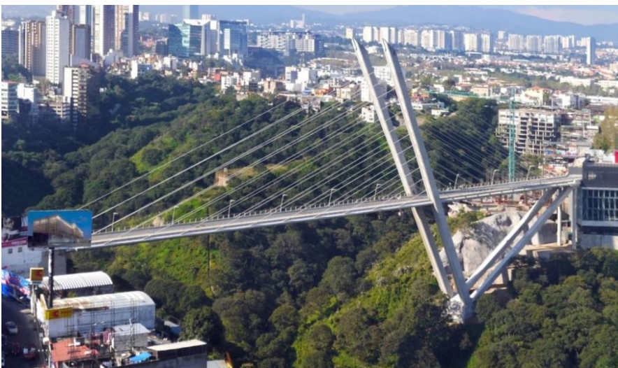
Fig. 4. General view of the bridge
