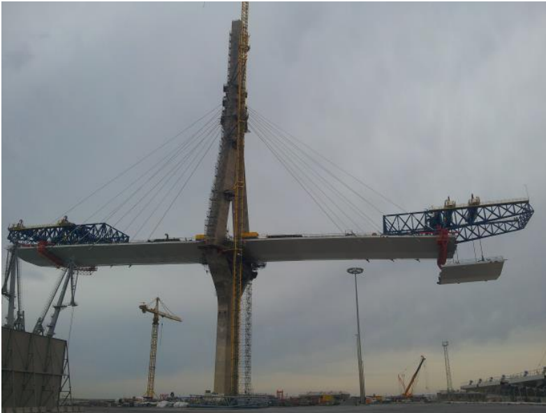
Fig. 5. Main span erection
