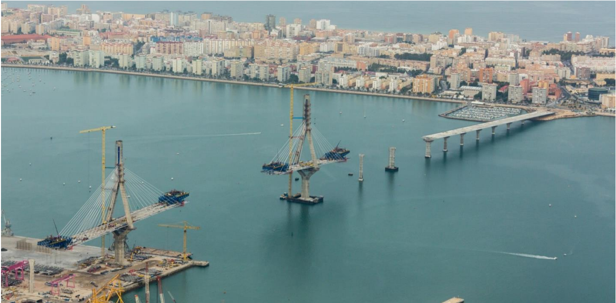
Fig. 1. General view of the bridge
