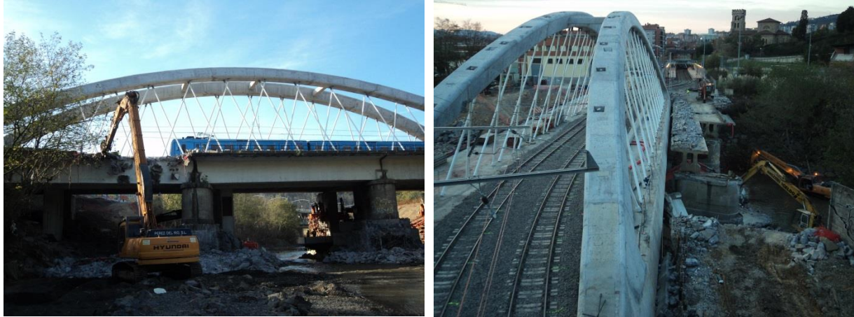
Fig. 7. Demolition of the existing structure
