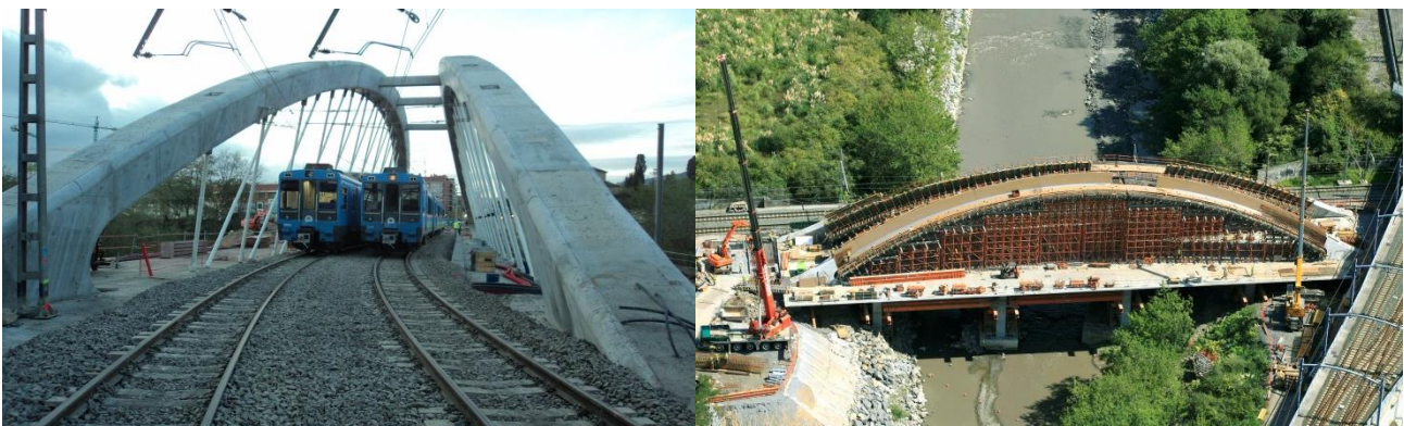
Fig. 5. Provisional tracks over the bridge
