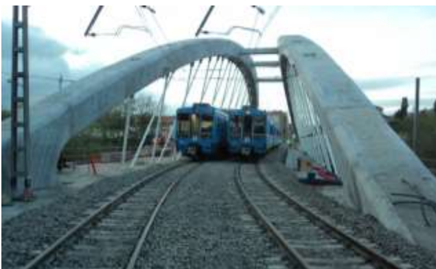
Fig. 5. Provisional tracks over the bridge
