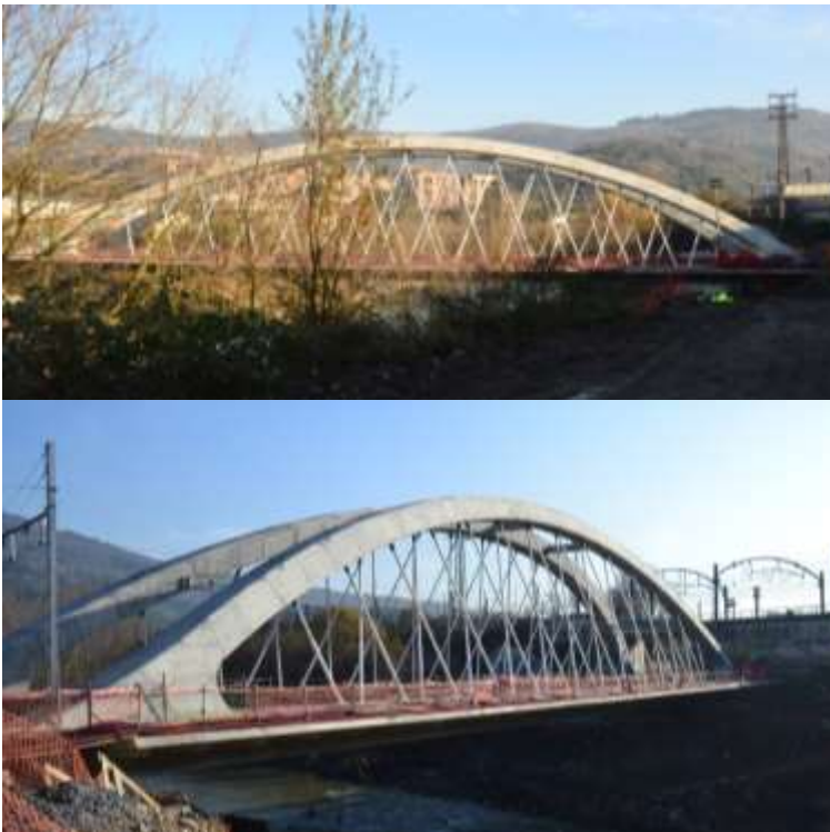
Fig. 4. General view of the bridge.
