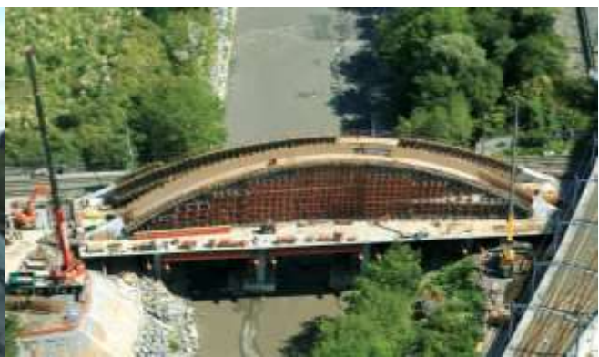
Fig. 6. Construction of the arch using a formwork
