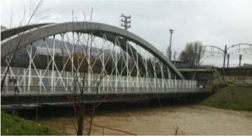
Fig. 2. Bridge with river at its highest level
