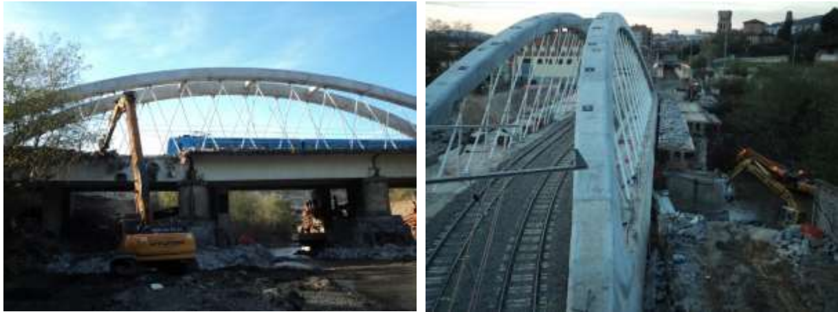
Fig. 7. Demolition of the existing structure
