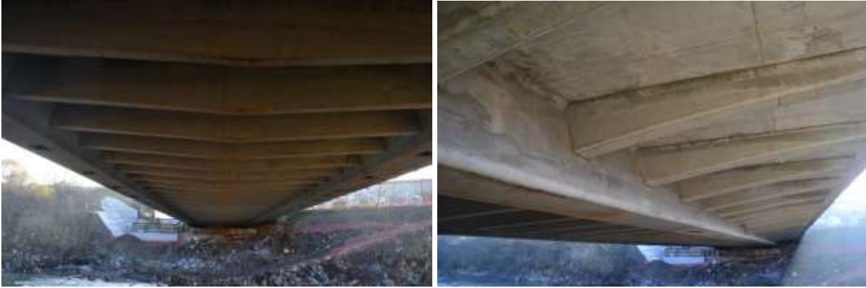
Fig. 5 Lower view of the deck
