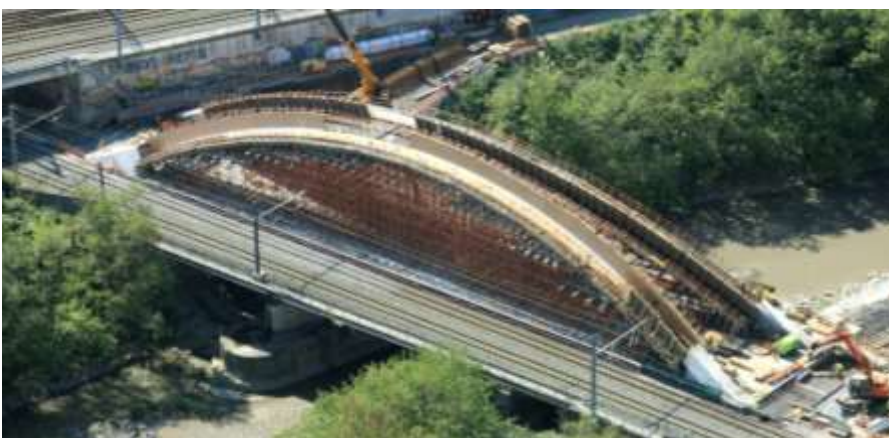
Fig. 3. Construction of the bridge parallel to the existing bridge
