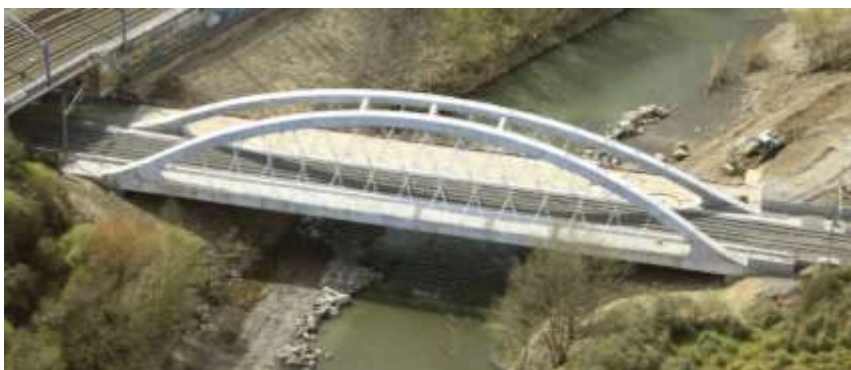
Fig. 1. Aerial view of the bridge
