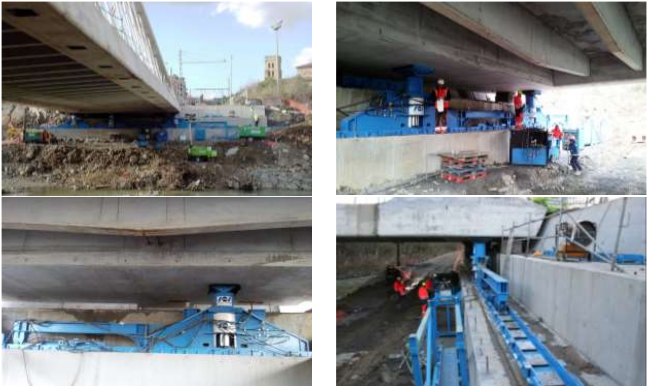
Fig. 8. Jacking and sliding of the bridge. Skid shoes and tracks
