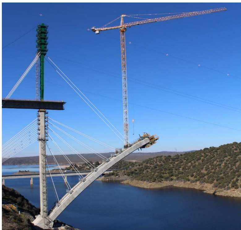
Fig. 4: Crane over the segment number 20 in its position number 2. The 7th stays pair is next to the crane. The first sixth couples are anchored to the pile.
