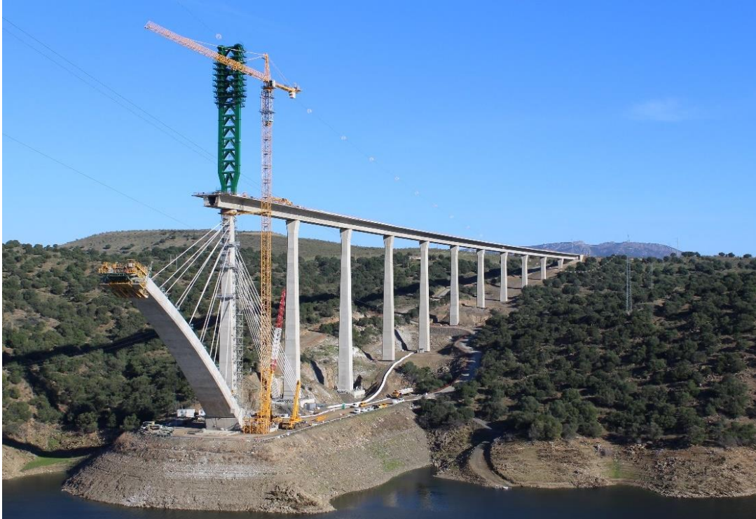
Fig. 2: The crane is put down to be moved to the position 2 (over the arch).
