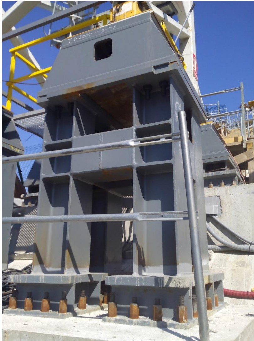
Fig. 6: Docking structure of the crane 1 on the arch.
