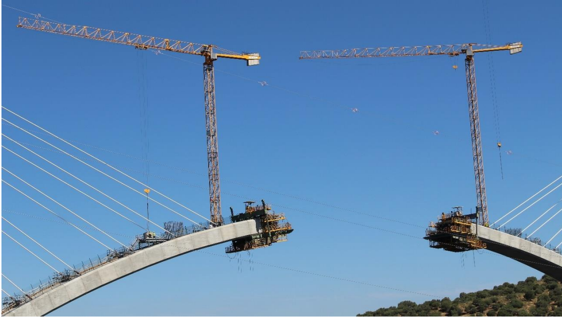
Fig. 5: Cranes 3 and 4. The left crane is placing loads in the material exchange platform. There are some operators on the platform.
