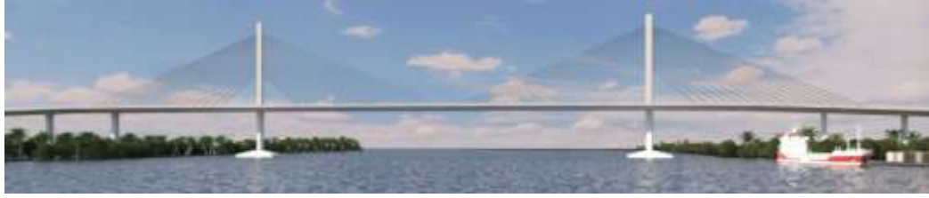
Fig. 3 Elevation and general view of the cable-stayed stretch.
