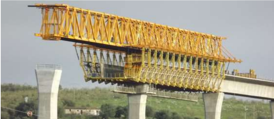
Figure 4. Deck construction with scaffolding truss
