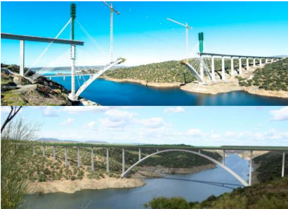
Figure 6. Current status / Final view of the bridge
