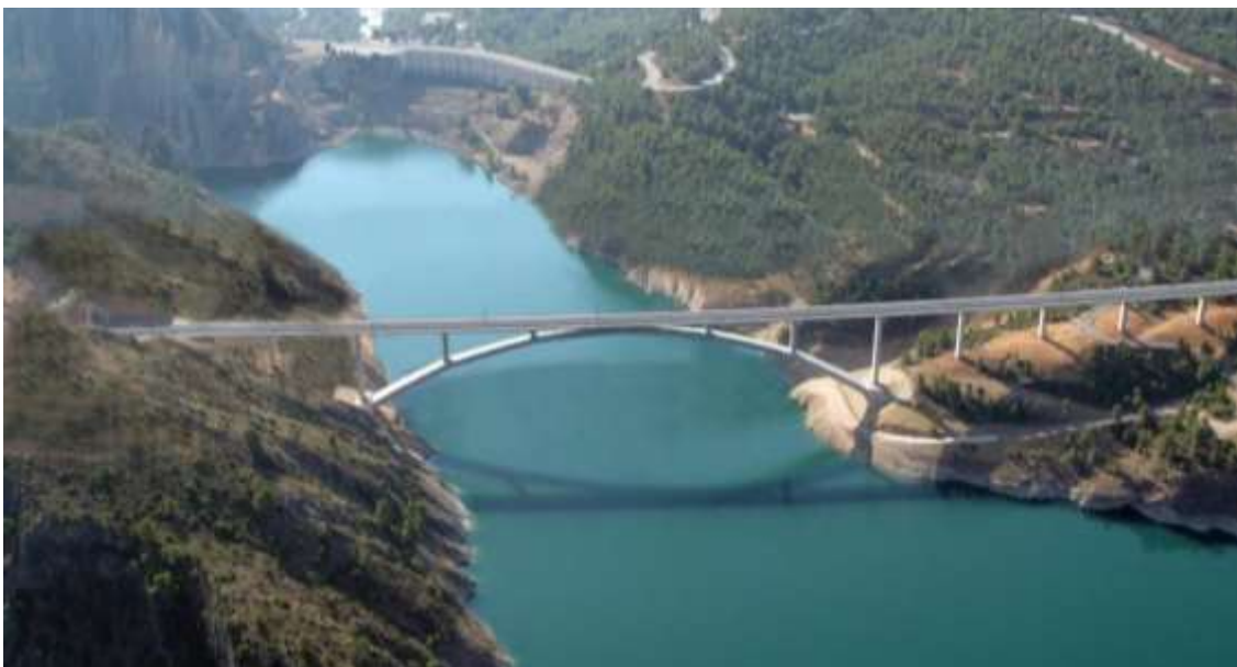
Figure 1. View of the arch bridge built over the Contreras Reservoir
