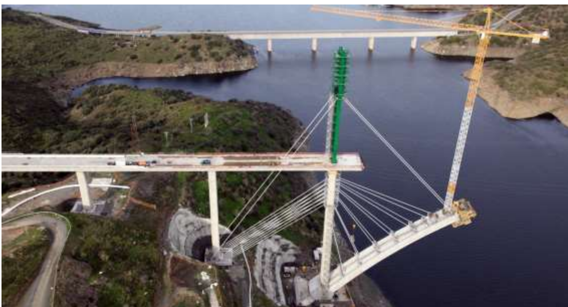
Figure 5 Arch erection with form traveler
