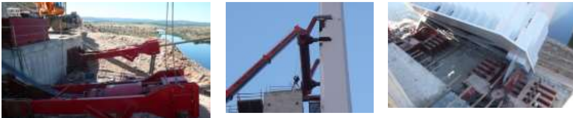
Figure 11. Retention hydraulic frame, auxiliary frame on the semi arch, provisional hunger
