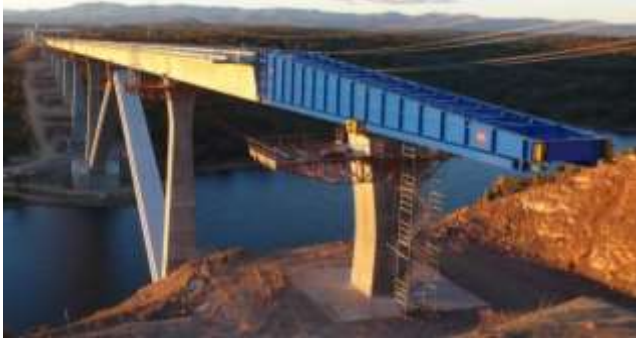
Figure 9. Launching nose
